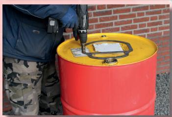
Place the washer of the front plate in the center of the barrel. Then drill the holes.
